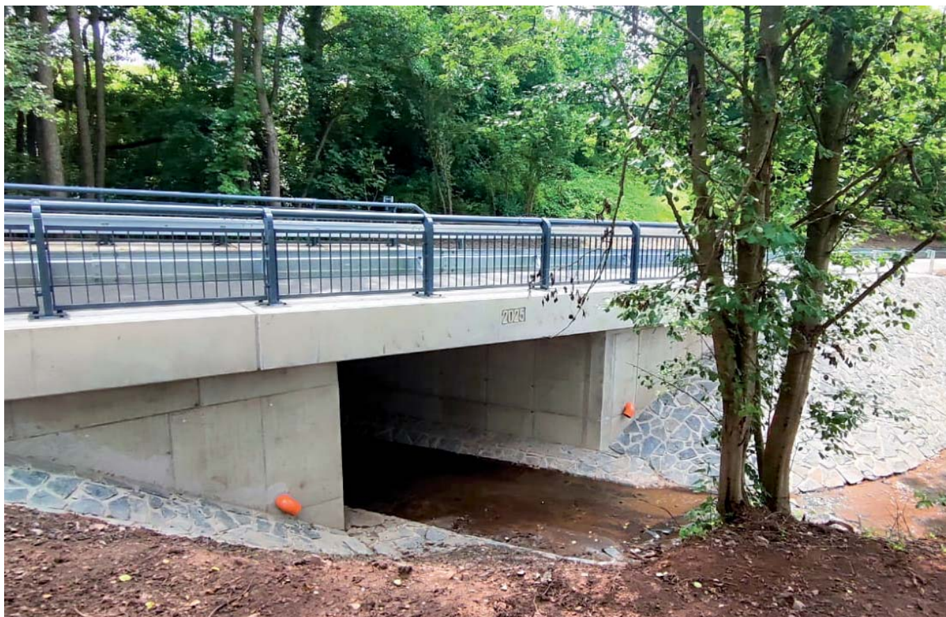
Most ev.č. 2836-1 Veselá
